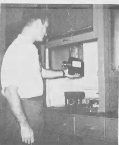
ERE'S INDUSTRIAL hygienist Richard S. Brief measures ventilation of laboratory hood with a device known as a Velometer.
